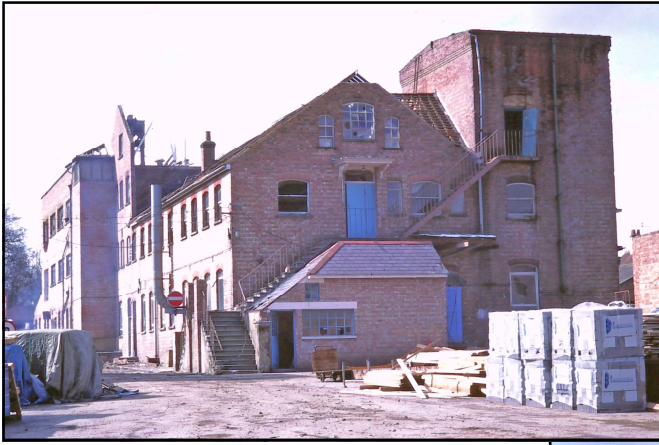
Left and below: Demolition of the Granose building
