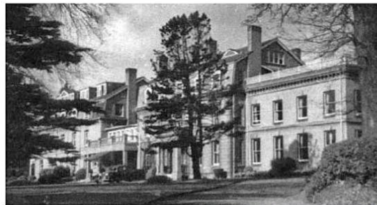
On 9 May 1912, the mansion on Stanborough Park, after considerable extensions, including two additional floors (which had once housed the college), was opened as the Stanborough Park Hydro. This was how the front of the building looked in 1938 after further significant development had taken place
