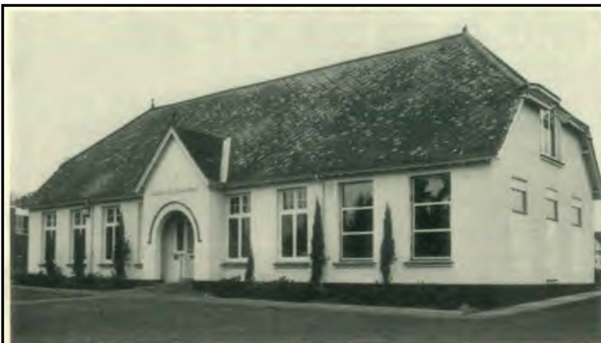
In addition to updating equipment in the radio studio at Stanborough Park, considerable renovation work has been undertaken. This has included the 'bricking-up' of several windows for security purposes; the installation of double- and treble-glazed windows for sound insulation; and a remodelling of the recording studio and control room which have remained unchanged since the inauguration of our British radio ministry in 1947. This year's radio offering will meet the cost of completing this constructional work, and the development of radio cassette, and video programmes to enlarge and enhance the communication of the Church's message.
